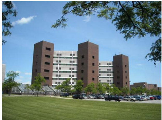
UB Cooke Hochstetter wet lab building with 200 fume hoods and 300,000 cfm of continuous outside air ventilation. Annual energy bill: $1,000,000+ (Photo credit: Walter Simpson)
